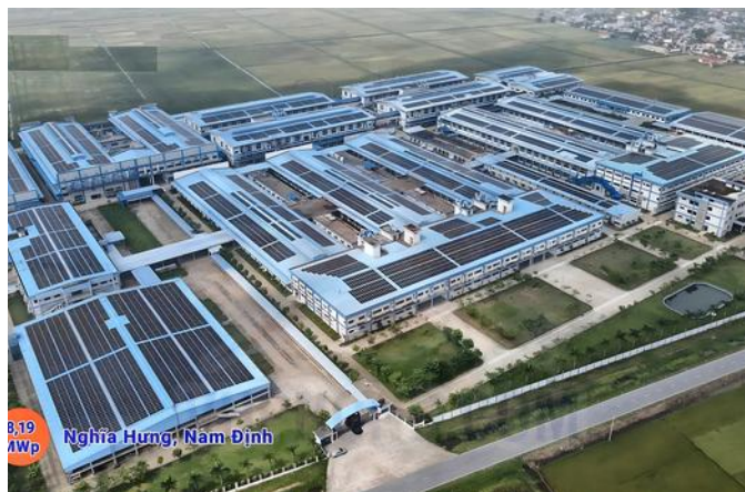
Golden Victory – Nam Dinh 8,190 kWp industrial rooftop · 2025
