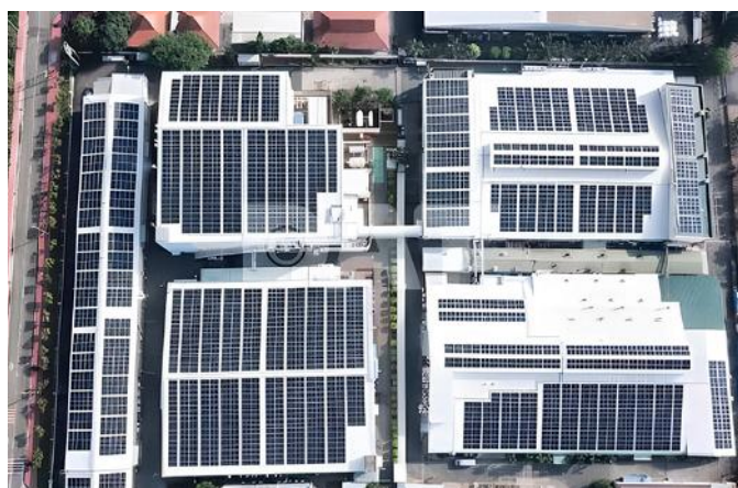
MEIWA Viet Nam – Binh Duong 1,700 kWp industrial rooftop · 2023
