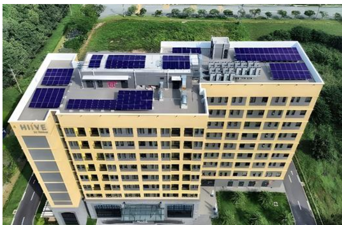
HHIVE Hotel – Binh Duong 85.2 kWp hybrid • 2024
