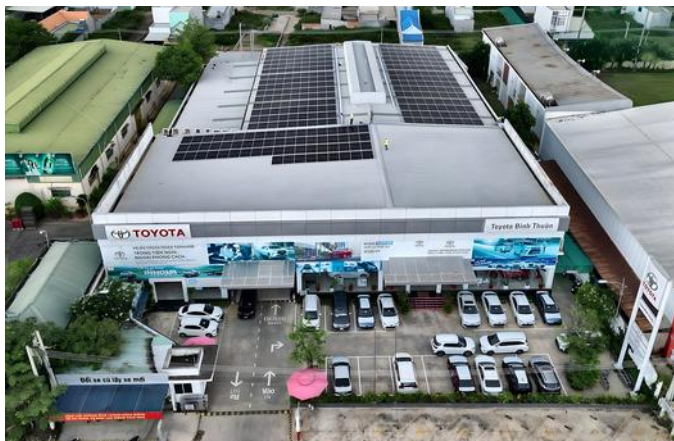
Toyota Binh Thuan 221 kWp commercial rooftop • 2023
