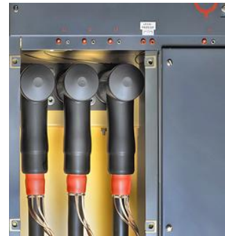
T-connectors on RMU bushings
