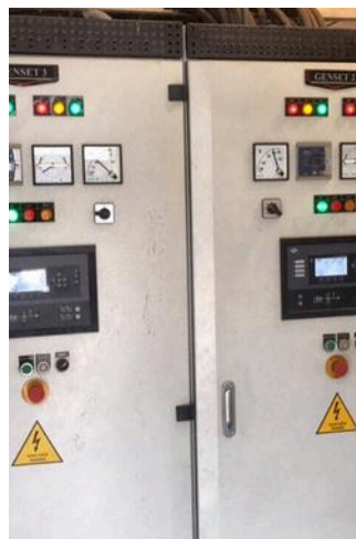
Generator synchronising switchboard – Shanghai Casino Resort (2018) ទូរសមកាលកម្មម៉ាស៊ីនភ្លើង – Shanghai Casino Resort (2018)
