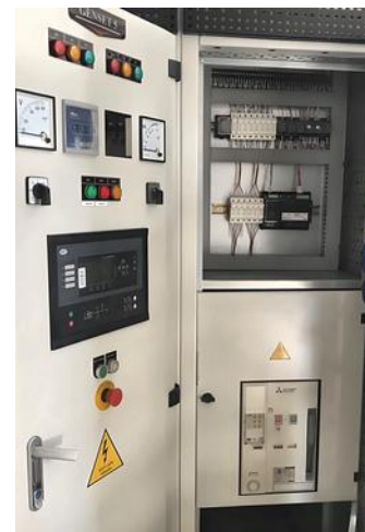
Generator synchronising switchboard – Shanghai Casino Resort (2018) ទូរសមកាលកម្មម៉ាស៊ីនភ្លើង – Shanghai Casino Resort (2018)
