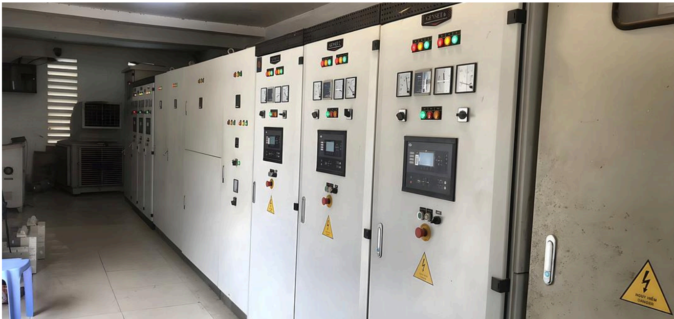
Generator synchronising switchboard – Shanghai Casino Resort (2018) ទូរសមកាលកម្មម៉ាស៊ីនភ្លើង – Shanghai Casino Resort (2018)
